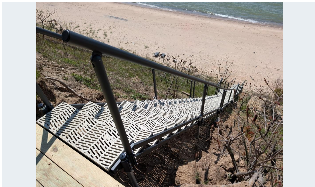
EZ Beach Steps adjustable aluminum stair system installed on a Lake Michigan bluff, providing adaptable access across changing shoreline and dune conditions. Photo courtesy of EZ Beach Steps.
